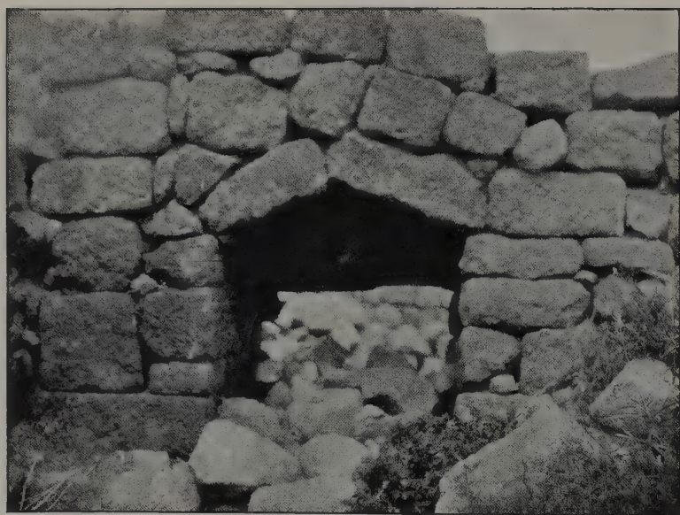
FIG. 237.—Village fort, interior of door in chamber of bastion.
